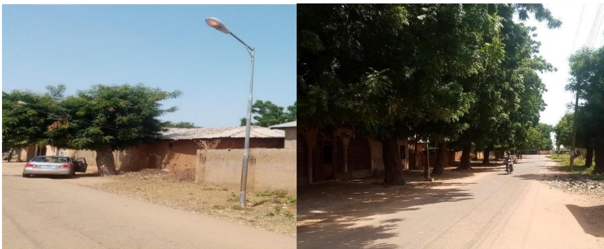
Plate 4. 11: Typical roads in Wamakko town
