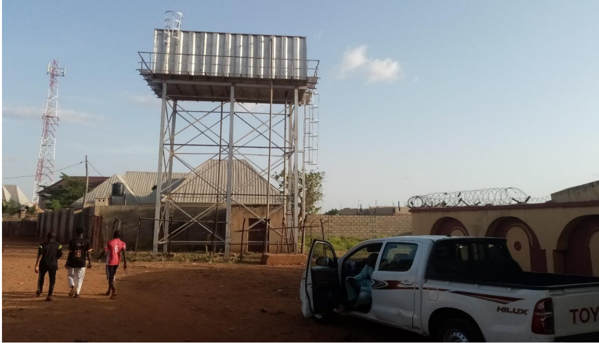
Plate 4. 9: A Motorized borehole in Sokoto
