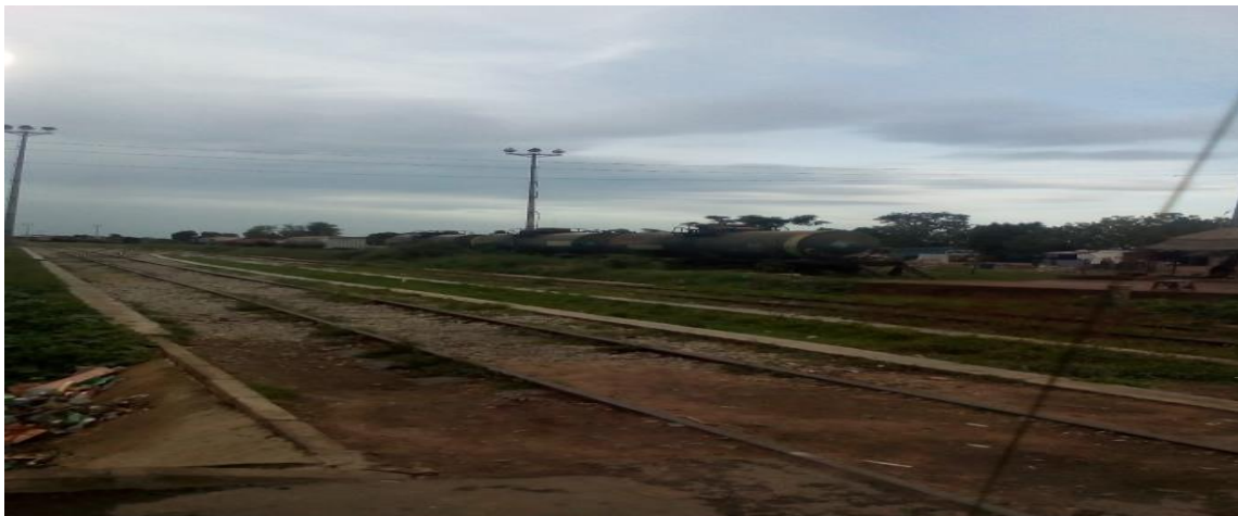
PLATE 3. 1 Abandoned rail transportation system
